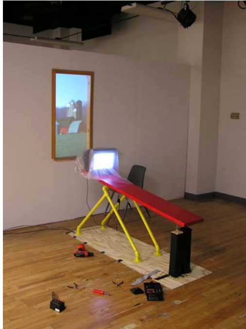
Educational Development, 2007. Framed-out recessed window and see-saw apparatus. Note black blocks for sensors and cables running under constructed wall.
